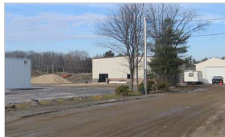
Existing Structure and Adjacent Land
